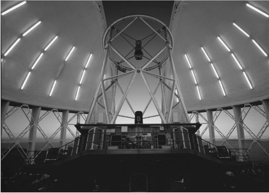
Figure 7.18: A view of the interior of the Gemini North telescope enclosure at sunset showing the fully open thermal vents and the fully open observing slit. (Courtesy of the International Gemini Observatory.)
